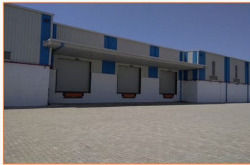
Loading Bays - Docks with levellers
