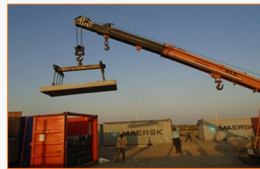
Open Yard for ODC and Container Ops
